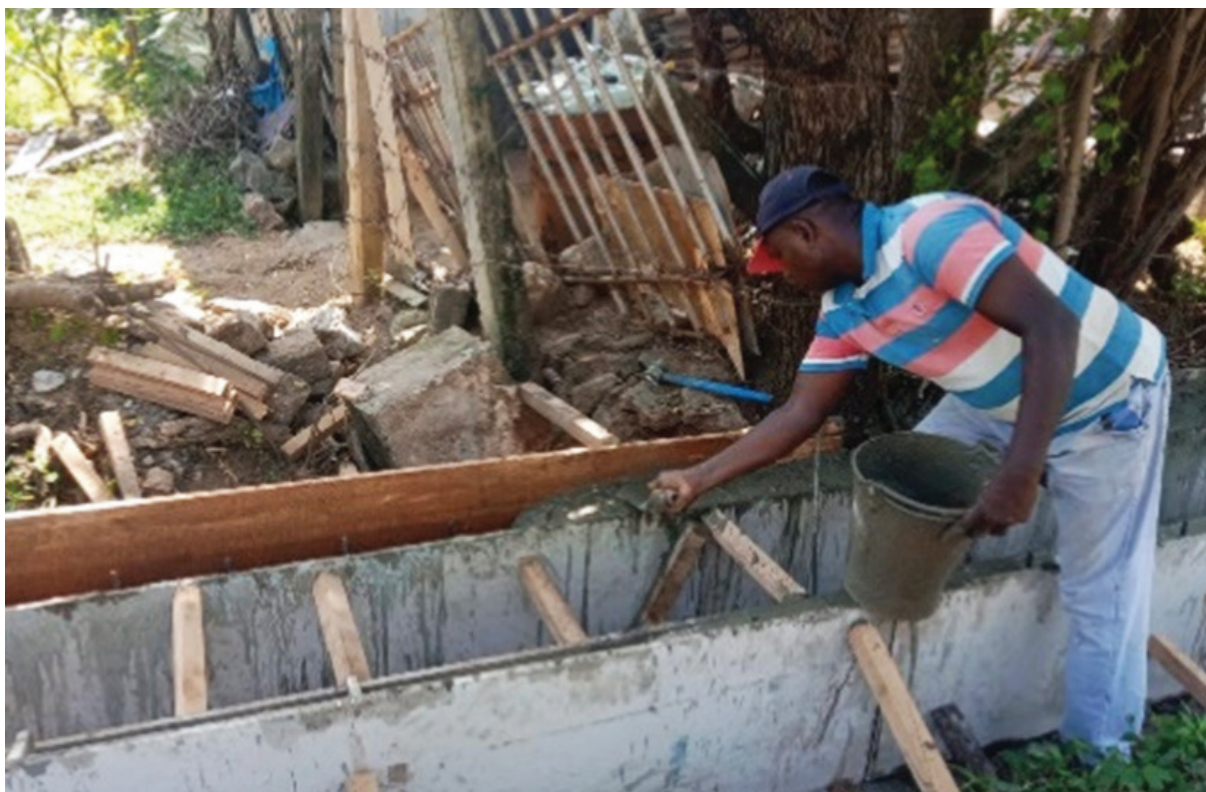
Construction of the drains in Abhayapura, Trincomalee.
